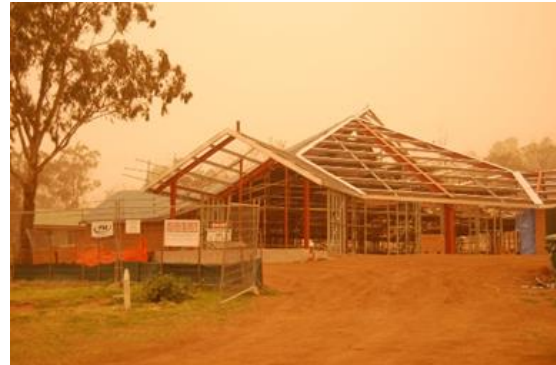
Fairfax Centre building works in a dust storm 2008
